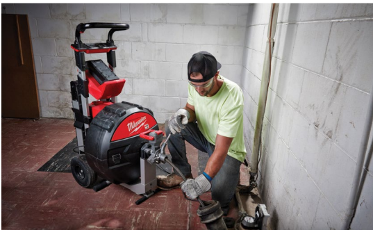
Sewer calls simplified
